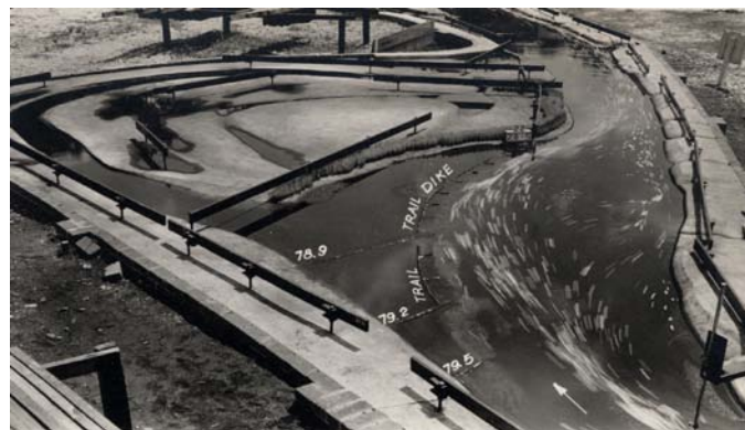
Railing system for large-scale coal bed models (U.S. Army Engineer Waterways Experiment 1937).
